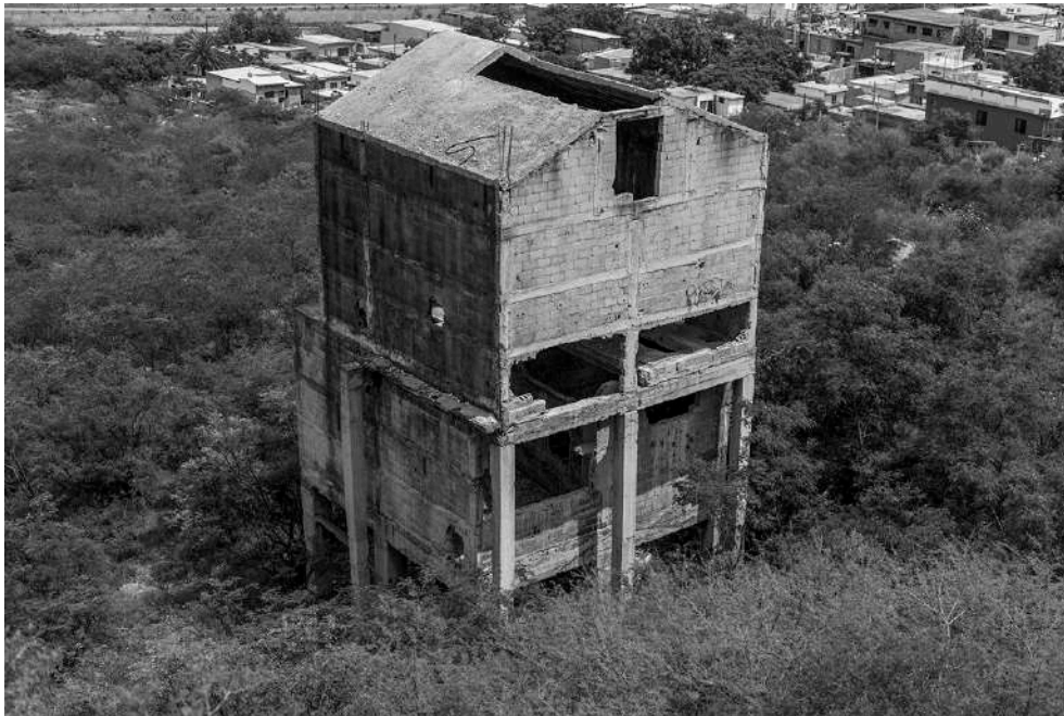
Figure 8: These old quarries still have the functional structures in which the crushers, conveyor belts and hopper were housed.
